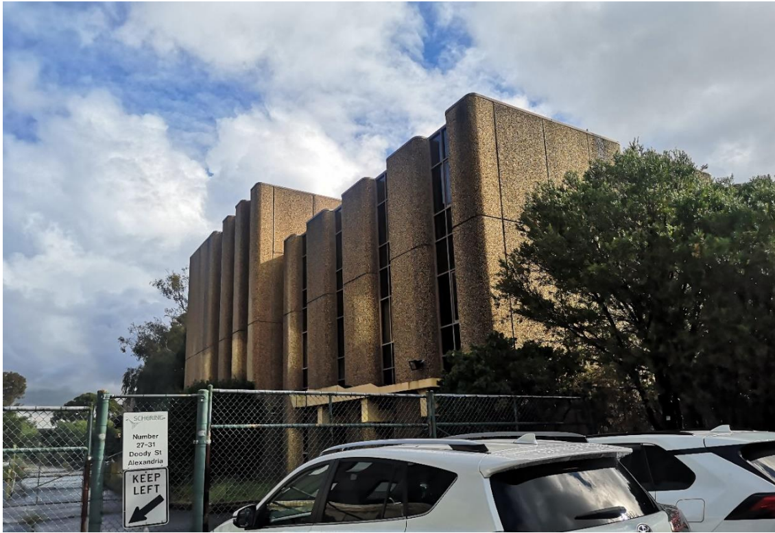
Figure 2: Site viewed from Doody Street looking south
