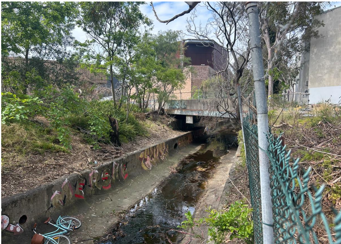
Figure 5: View of the open channel looking east towards the eastern boundary
