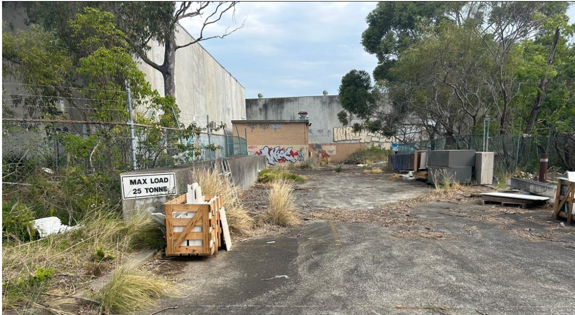
Figure 4: View of the bridge over the stormwater channel looking south towards the southern boundary
